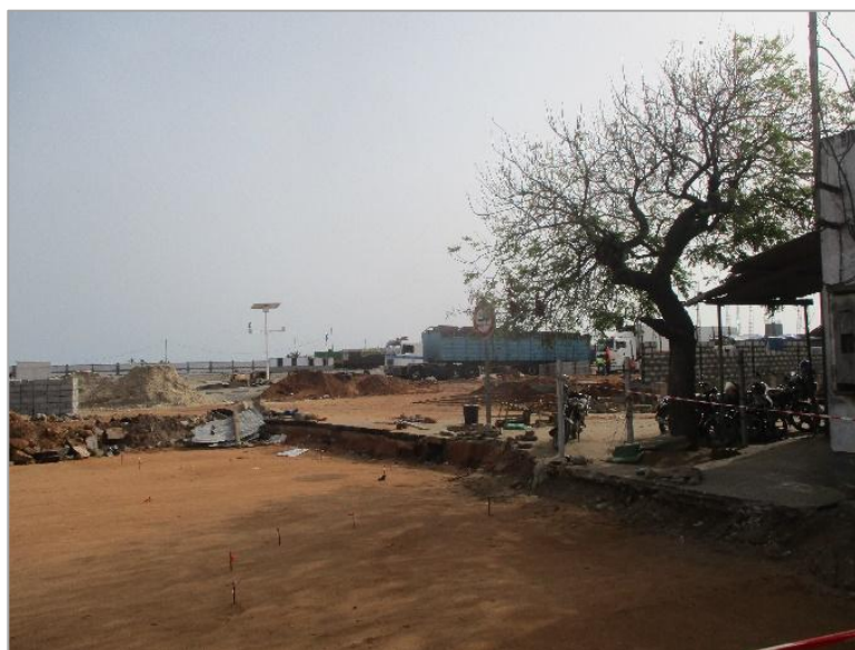
Photo 4: Demolition and reconstruction operations at the Sanvée-Condji/Hilla-Condji OSBP at the Togo/Benin border
