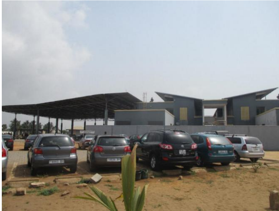
Source: DJOLAR Kossigari, Sanvée-Condji, October 13, 2020 Photo 3: The northern administrative block of the Noépé/Akanu OSBP
